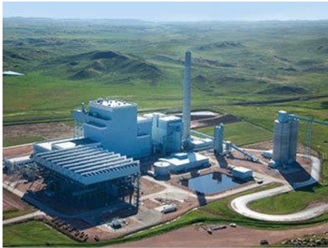
Located 7 miles north of Gillette, the Dry Fork Station quickly rises into view out of the hilly landscape.
